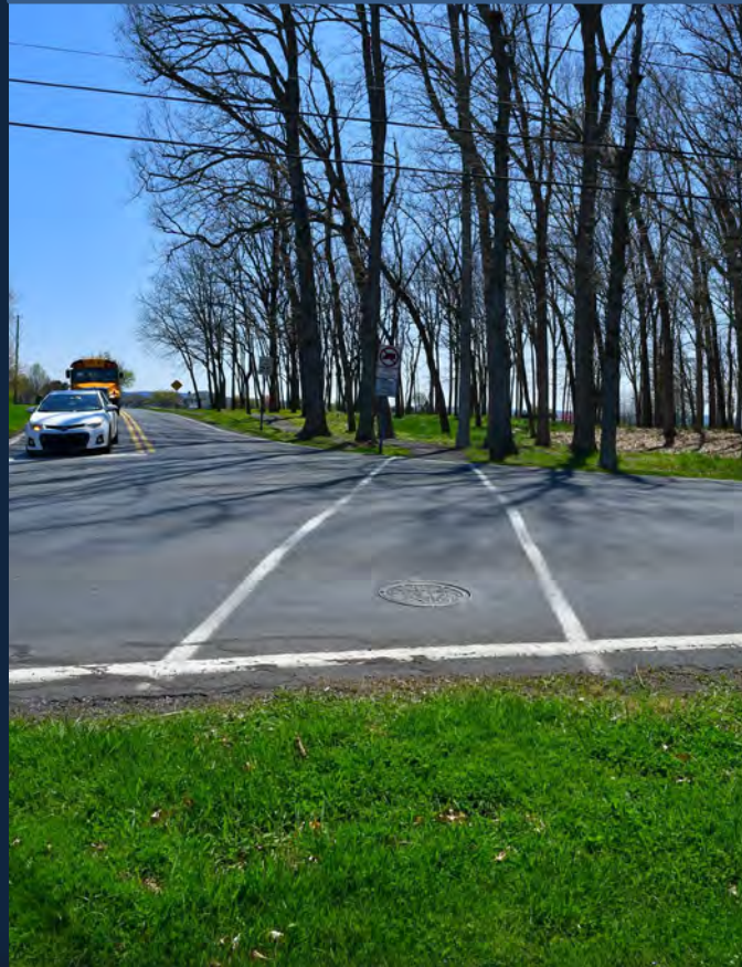
Existing Crosswalk: Schantz & Lone Lane Park
